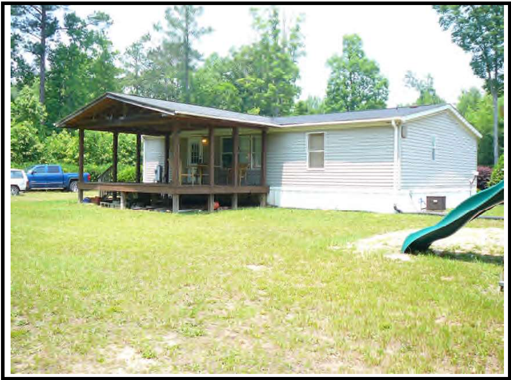
#4 – View the Manufactured Home (To be Razed) on the Subject Property Taken By Cedar Creek Appraisals 6/8/2023
